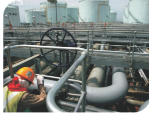
Water Piping System
